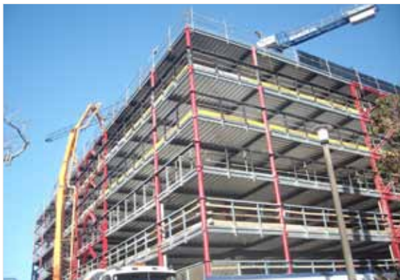
Pumping the KIM-treated concrete to level seven of the parking structure.
