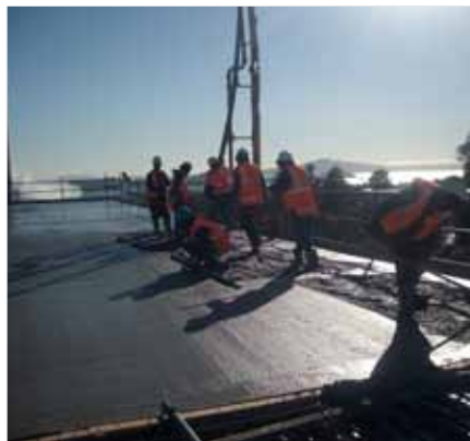
Finishing the concrete slab roof.
