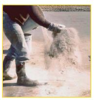
Krystol Broadcast produces a smooth finish and is used to integrally waterproof and add durability to concrete slabs that will be power-troweled during finishing:
